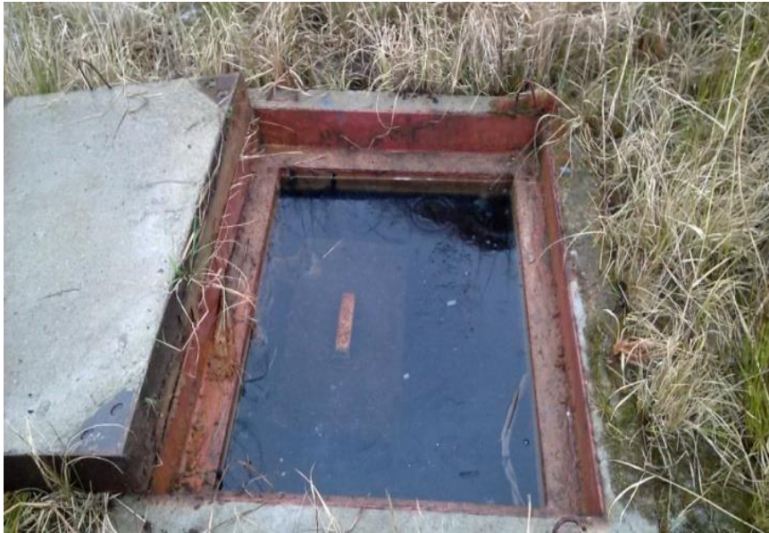
Photo 2. A concrete well filled with water.
