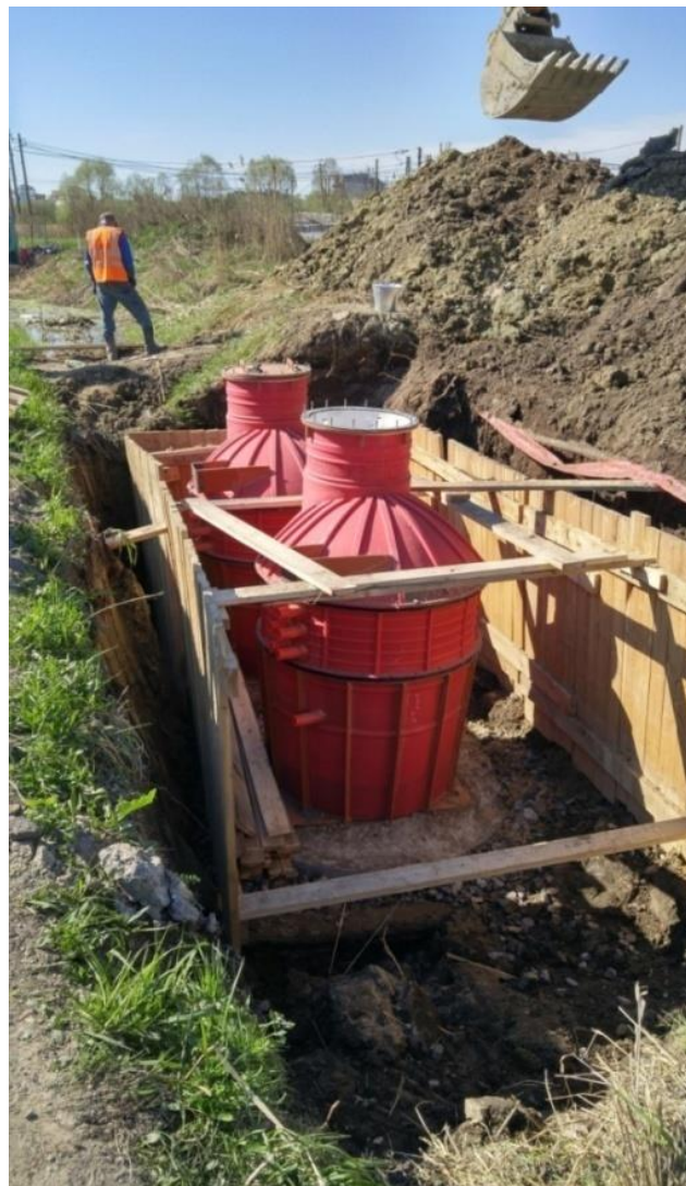
Photo 1. Installation of polymer wells for link-boxes.
