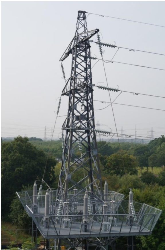
Fig.6. TP on the OHL tower having a platform for equipment covered with a grid: (a) – lattice; (b) – steel pole
