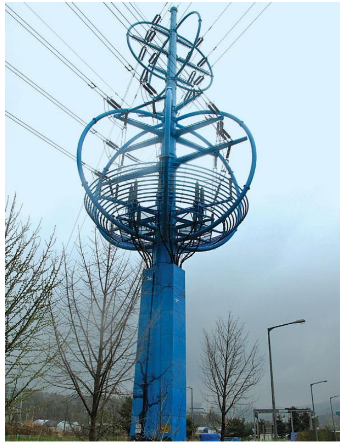
Fig.6. TP on the OHL tower having a platform for equipment covered with a grid: (a) – lattice; (b) – steel pole
