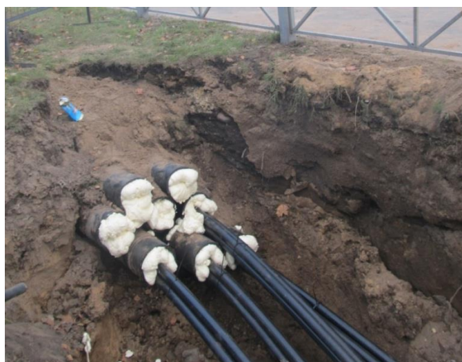
Fig.4. Unpainted pipe made of ordinary polyethylene. It does not have an internal nonflammable (NF) layer and seals (foam instead). The solution is designed for CL up to 1 kV.
