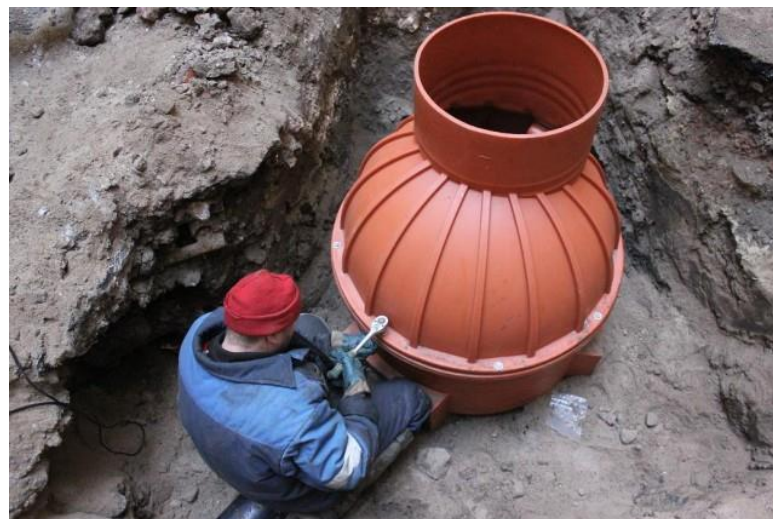
Fig.4. A fully plastic well with 100% tightness.
